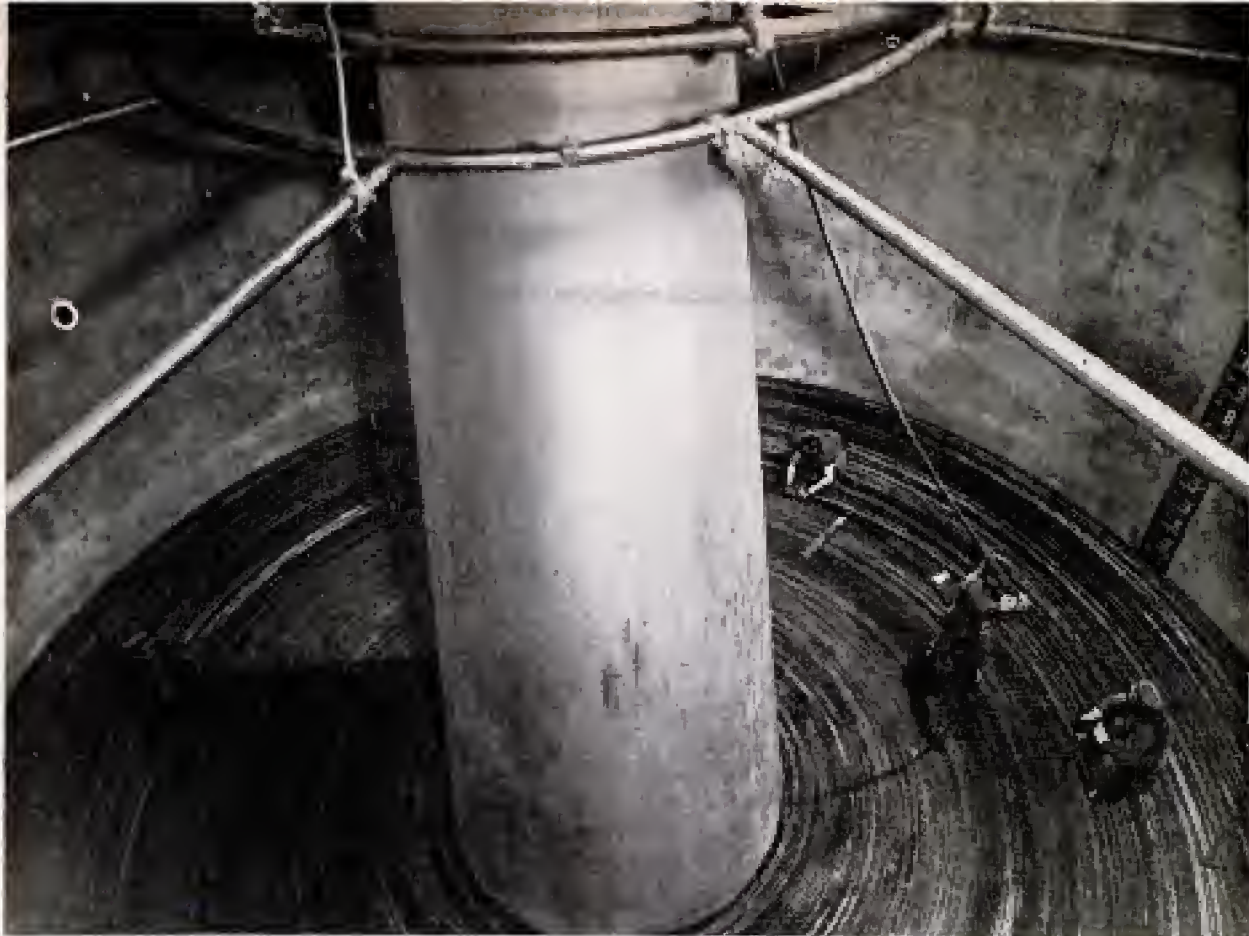
Careful loading of cable on ship takes weeks. Deep-water cable is 1½ inches thick, shallow cable is 2½ inches
